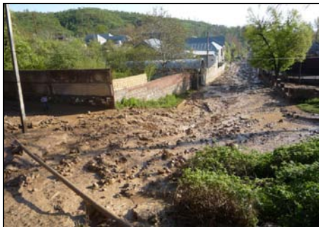
Picture 1. The motor roads of Gushchu-Zaylik were seriously damaged, some parts being washed down were fell into disrepair, 2009.
